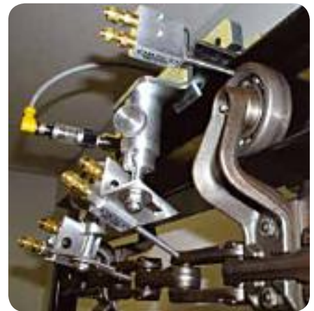
Image 1. Both the chain pins and wheel bearings on this overhead conveyor are being lubricated with four nozzles. A proximity switch times the intermittent spray to only lubricate the wear points.
