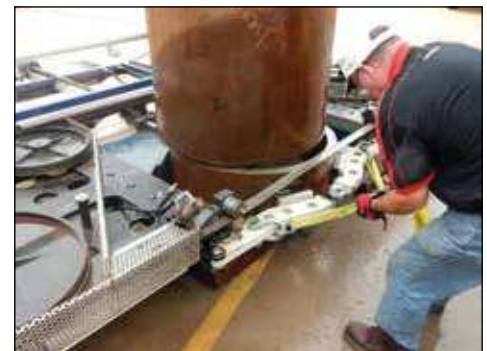
▲ Pipe cutting with BS portable band saw.
