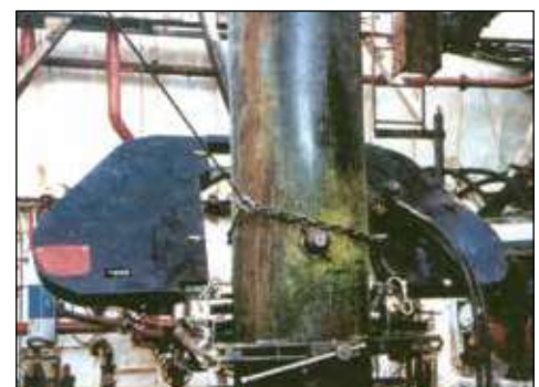
▼ Decommissioning job with band saw.
