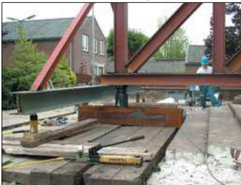
▼ P392 in action with RC256 cylinders.
