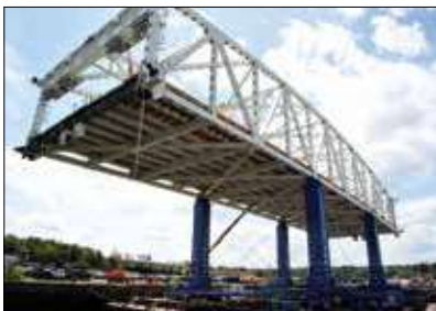
Incremental bridge lifting
