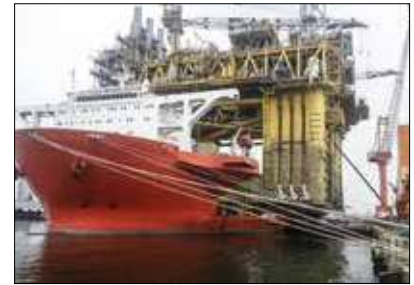
Synchronous superlift and launch
