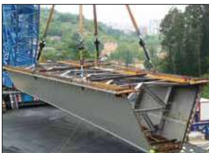
▼ Bridge segments are hoisted from the ground, being positioned with a 4-point SyncHoist system with fully monitored cylinders.
