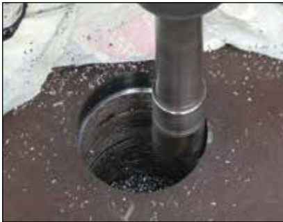
▲ Enlarging a hole
