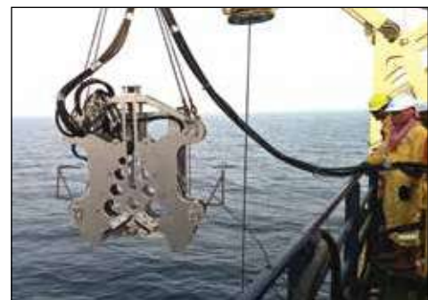
▲ MDWS Diamond Wire Saw lowered into sea.
