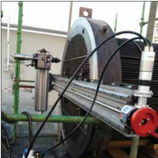
▼ MRY Milling machine on a heat exchanger.
