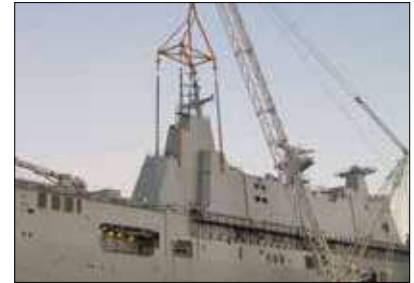
Synchronous hoisting and load positioning
