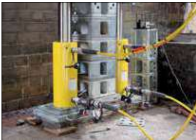
Bridge lifting and launching
