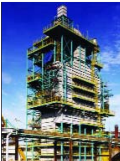
Ethylene Cracker Unit
