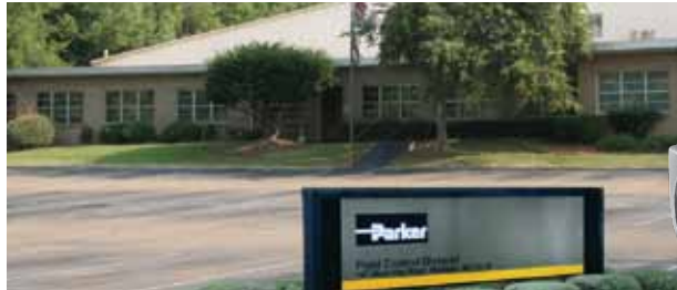
Fluid Control Division Facility, Madison, MS.
